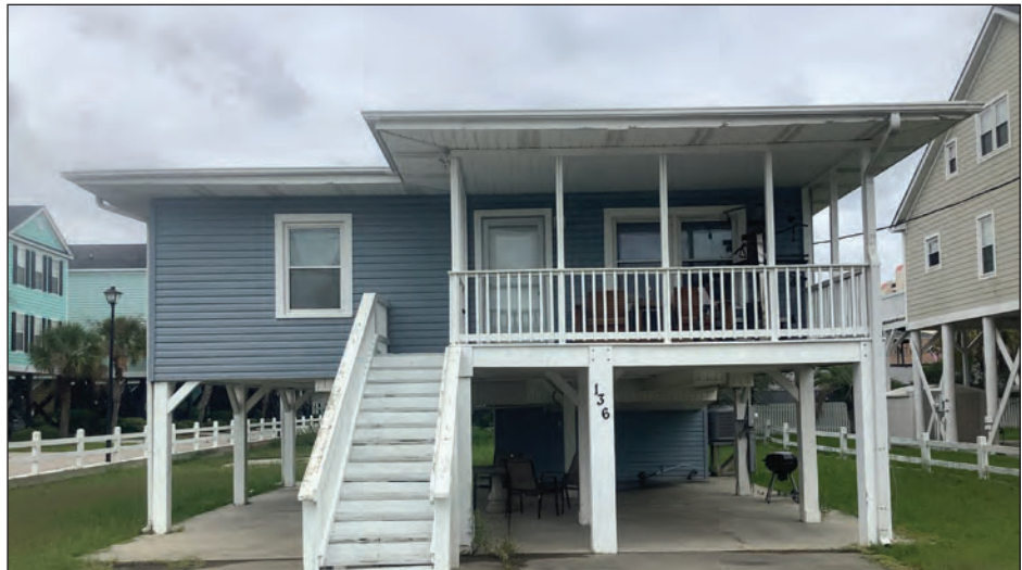
B. Façade, Facing Northeast
