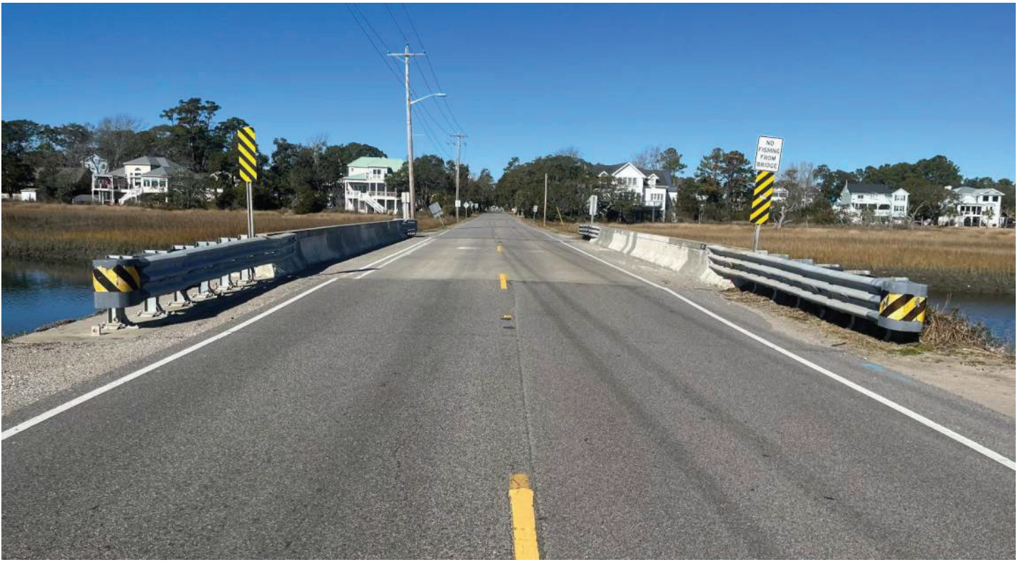
PHOTO # 1 View of the bridge facing northwest.
