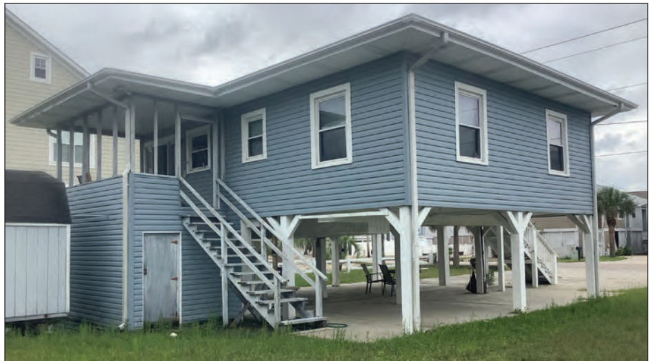
C. Rear Oblique, Facing South
