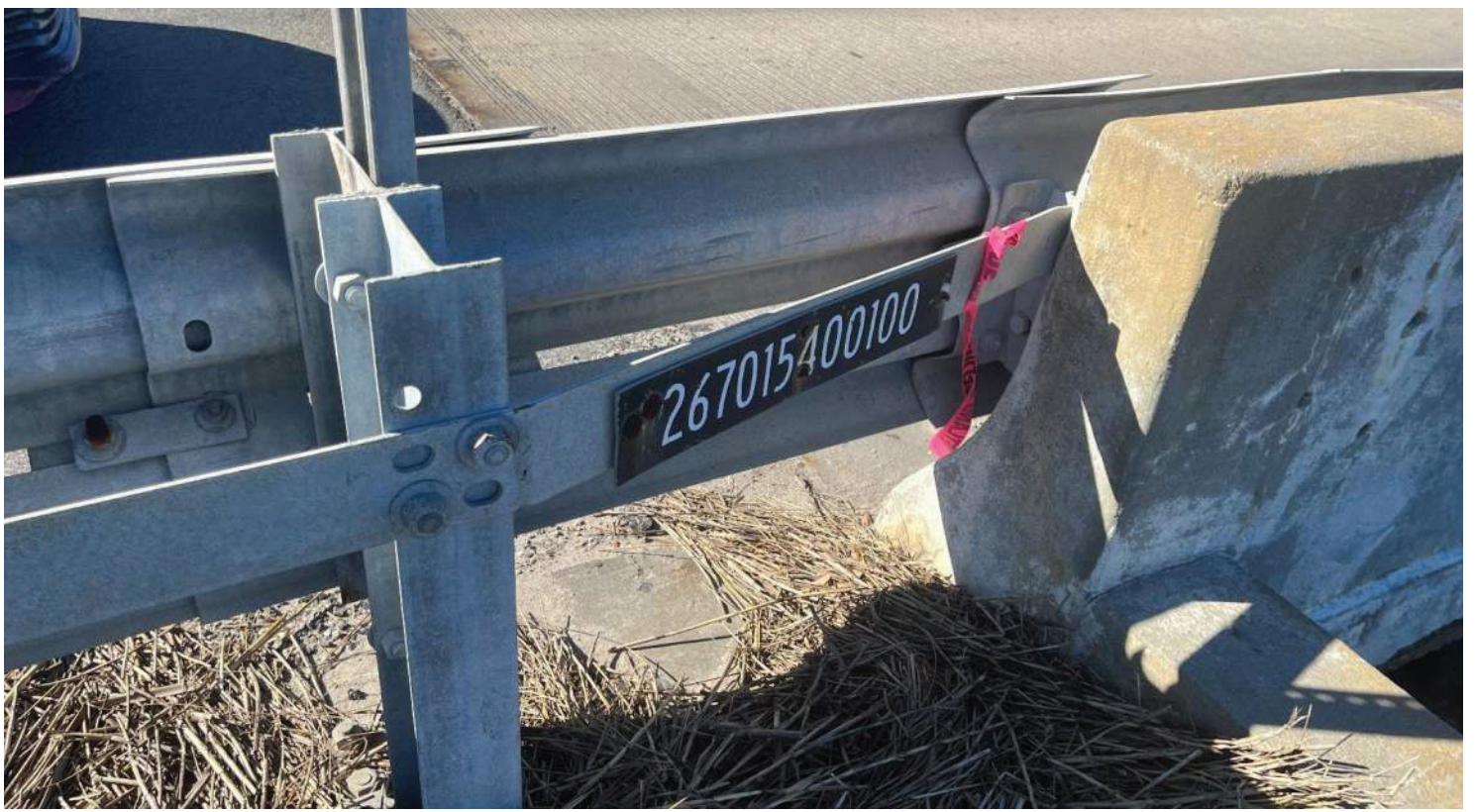
PHOTO # 3 View of the bridge number.
