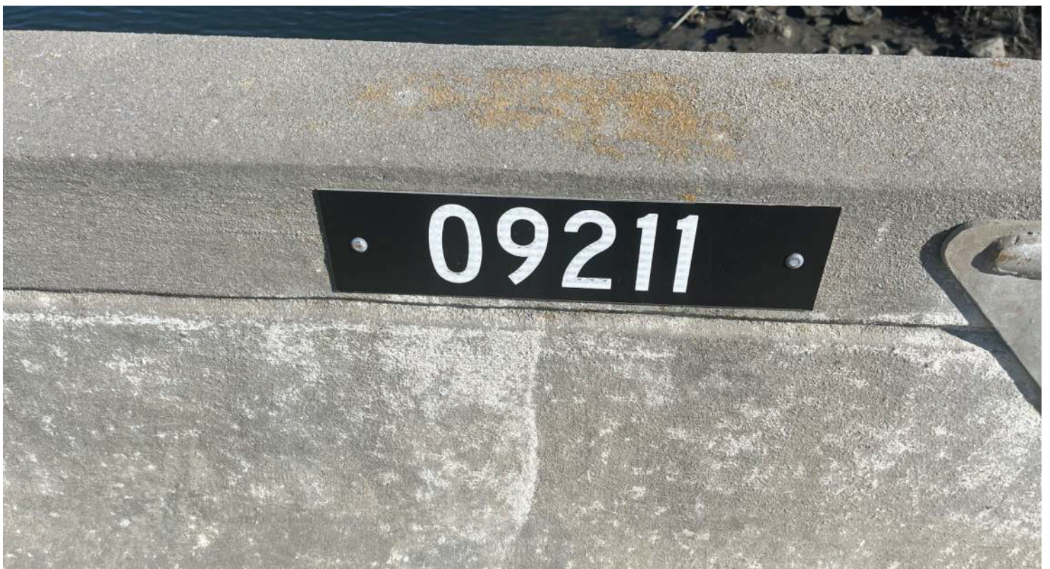
PHOTO # 4 View of the bridge asset number.
