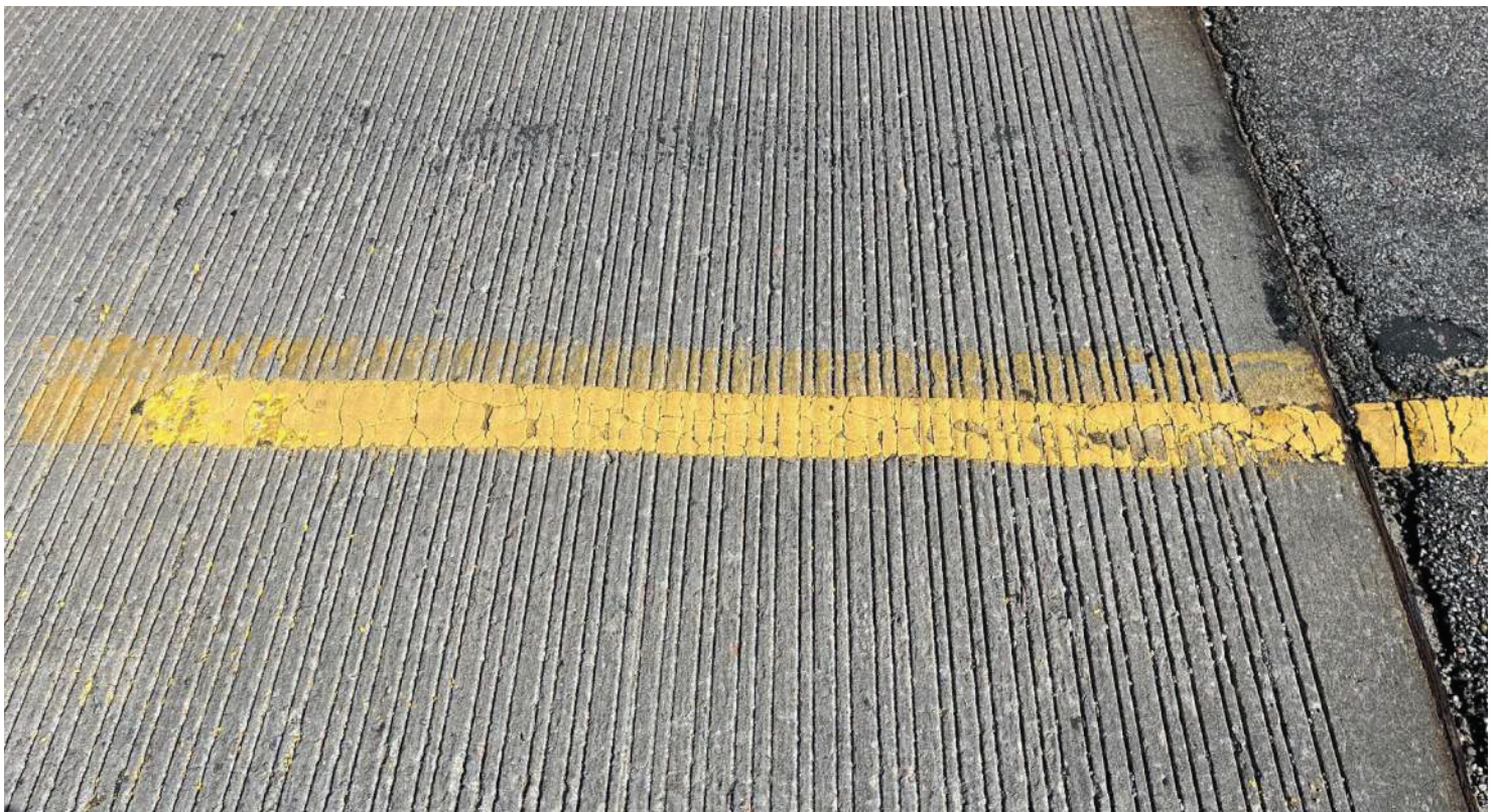
PHOTO # 8 View of LP-1 yellow line paint.
