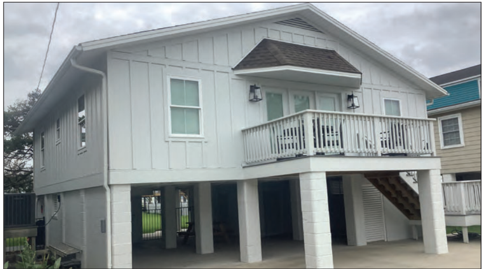
B. Oblique, Facing West
