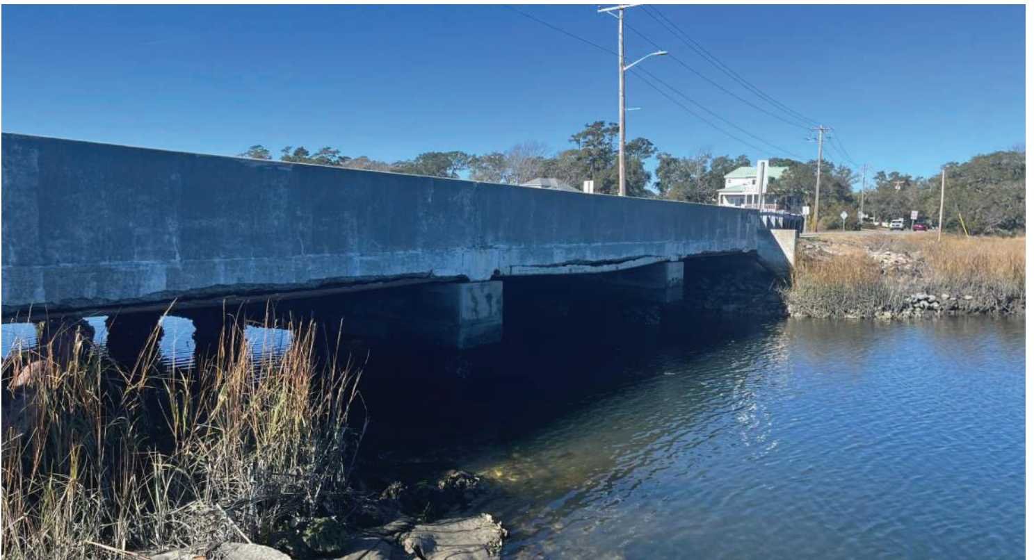
PHOTO # 2 View of the side of the bridge facing west.
