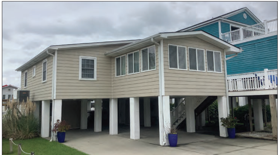
B. Oblique, Facing West
