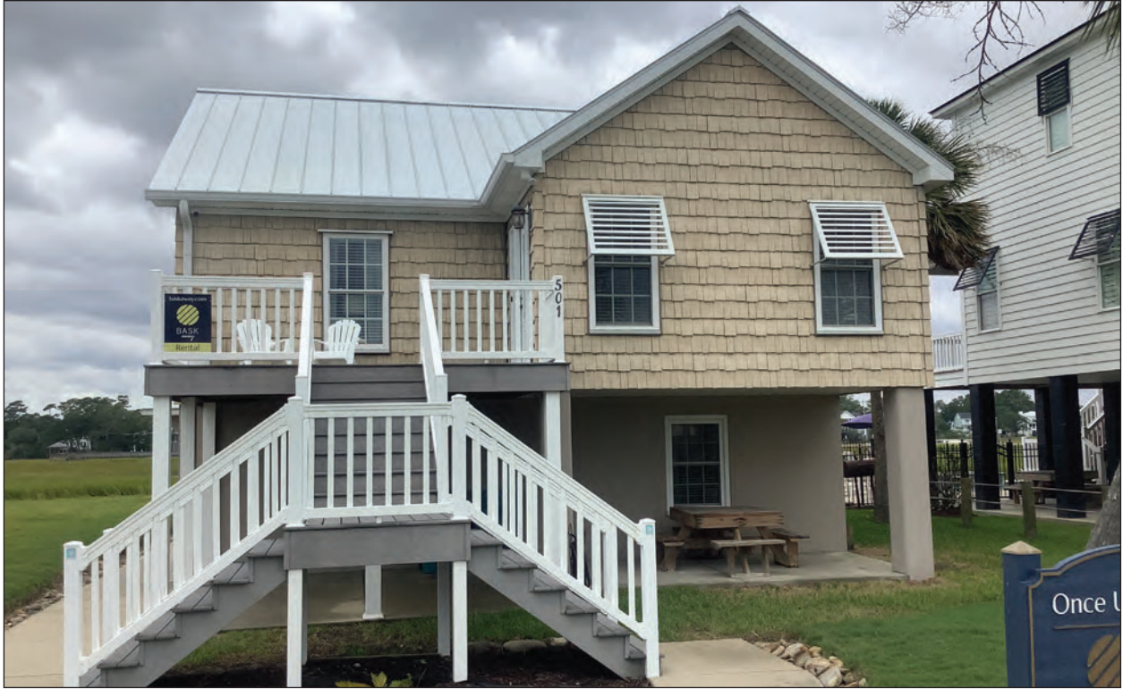
A. Façade, Facing Northwest
